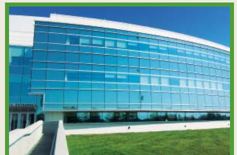
New Castle County Public Safety Building, New Castle, DE – LEED Silver
