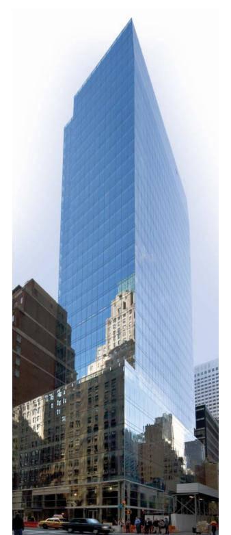
Invisiwall<sup>TM</sup> IGUs can be constructed with tempered glass using clear, low-iron, pyrolytic or laminated glass. The holes for the fittings are cut with our precision CNC fabrication machine.
