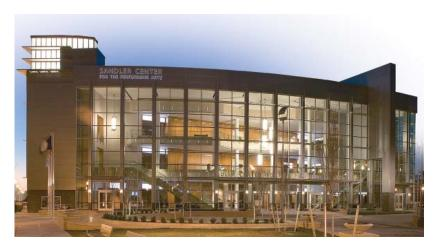
The argon-filled Winduo® IG units improve the insulating properties (reduce the U-Value) and improve the OITC (Outdoor Indoor Transmission Class) rating when used in place of air. The insulating units are filled with argon while being sealed without adding an entry gap in the spacer as in older methods. For quality assurance, the argon content can be accurately measured non-evasively using a Sparklike Gasglass instrument.
