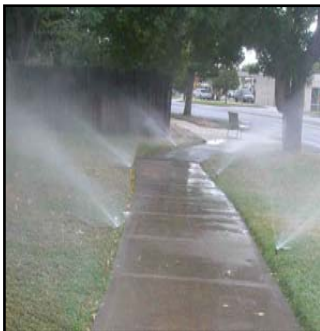
Overspray creates runoff and wastes water.
