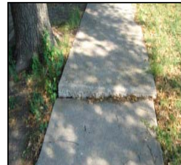
Surface roots have raised the sidewalk.
